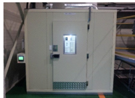
Fig. 3 Constant temperature and humidity room in Large Cavitation Tunnel (LCT) of KRISO
